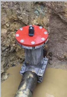
6 inch Insta-Valve 250 Patriot Series installed in Winchester, KY
